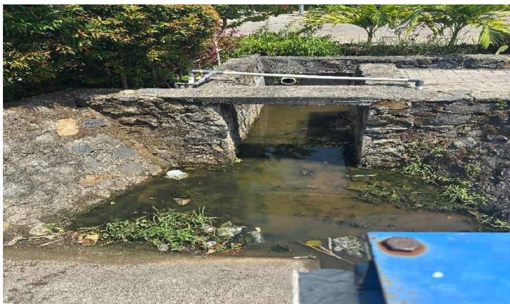
Channel Shelter from Impregnated WWTP Retention Pond
