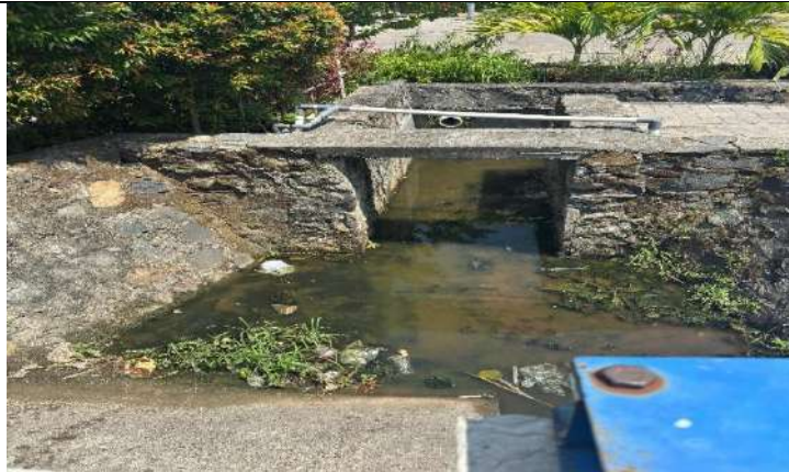
5. Integrated Waste Drainage and Treatment System in Each Campus Building
