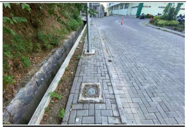
Use of paving blocks on every road section
