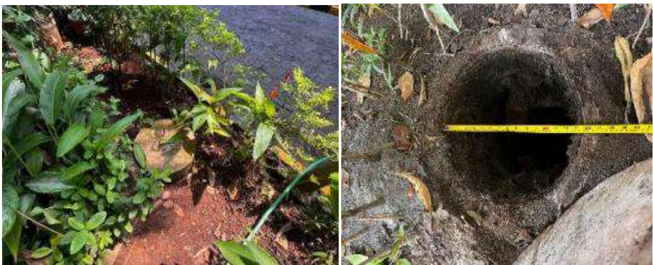
Preparation of Infiltration Wells
