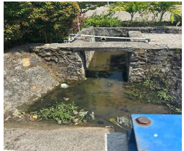
Channel Shelter from Impregnated WWTP Retention Pond
