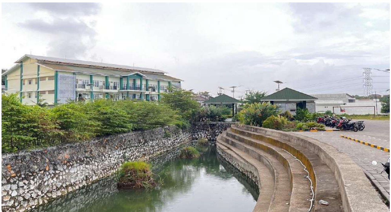
3. Reservoir of Rainwater Infiltration
