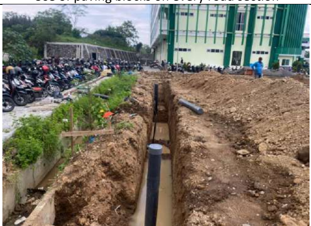
Preparation of Infiltration Wells
