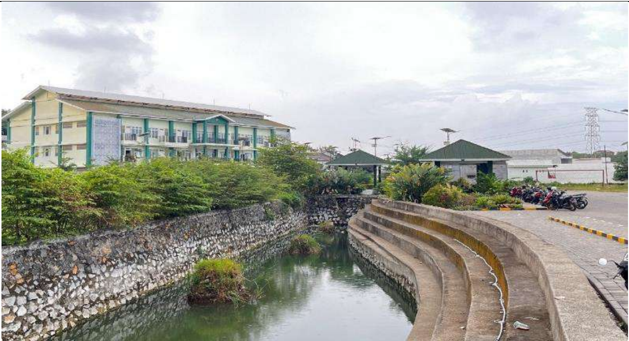
1. Construction of Infiltration Reservoirs and Rainwater Utilization
