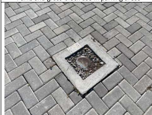
Preparation of Infiltration Wells
