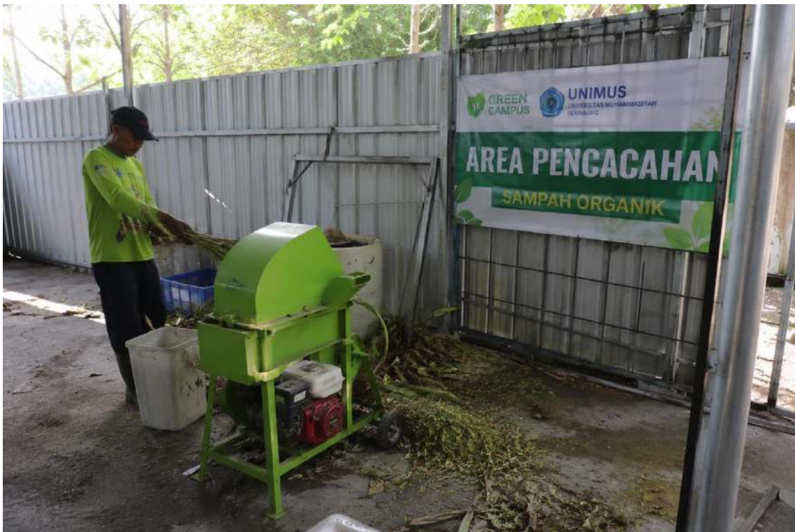
Waste Shredding Area
