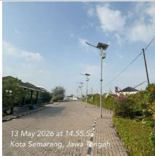
Solar Power Systems
