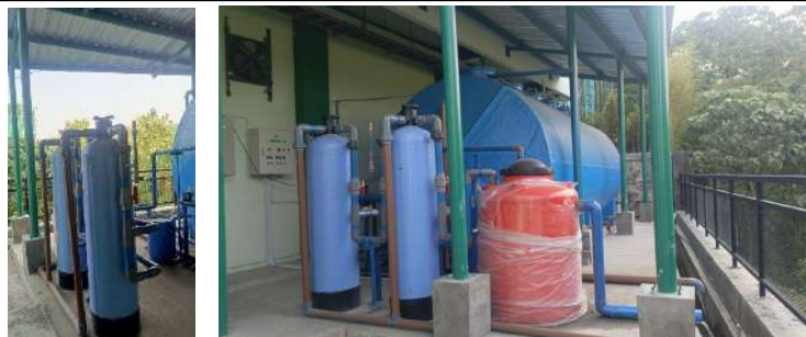
Water & Waste Energy Recovery (Waste-to-energy project)
