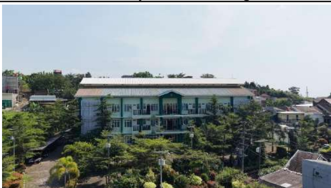
FTIK laboratory building
