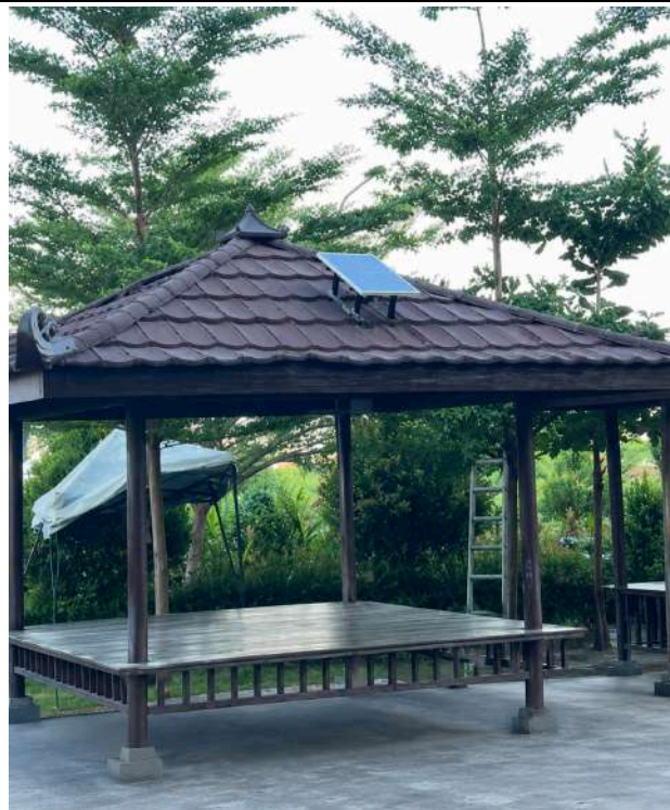
PLTS OFF GRID Gazebo Unimus
