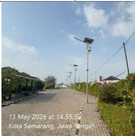
Solar Power (PJU)
