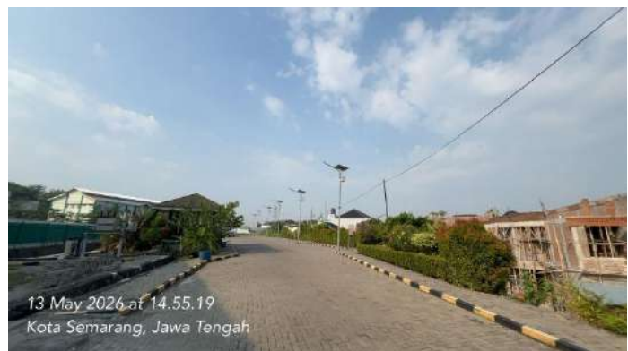
Solar Power (PJU)
