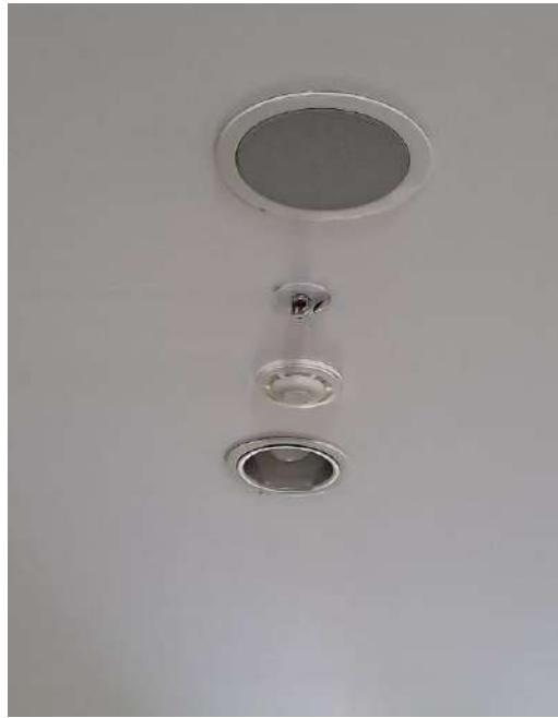
Smoke Detector, Springler and Speaker Paging
