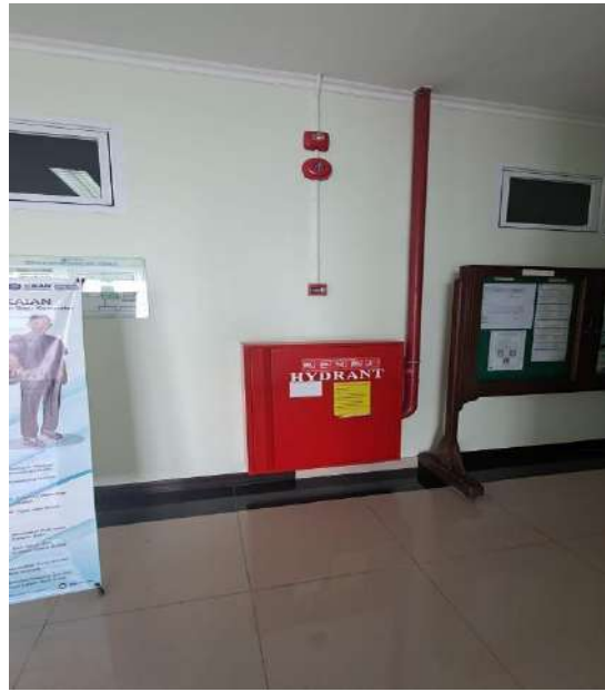
Fire Alarm and Hydran Box in the Building
