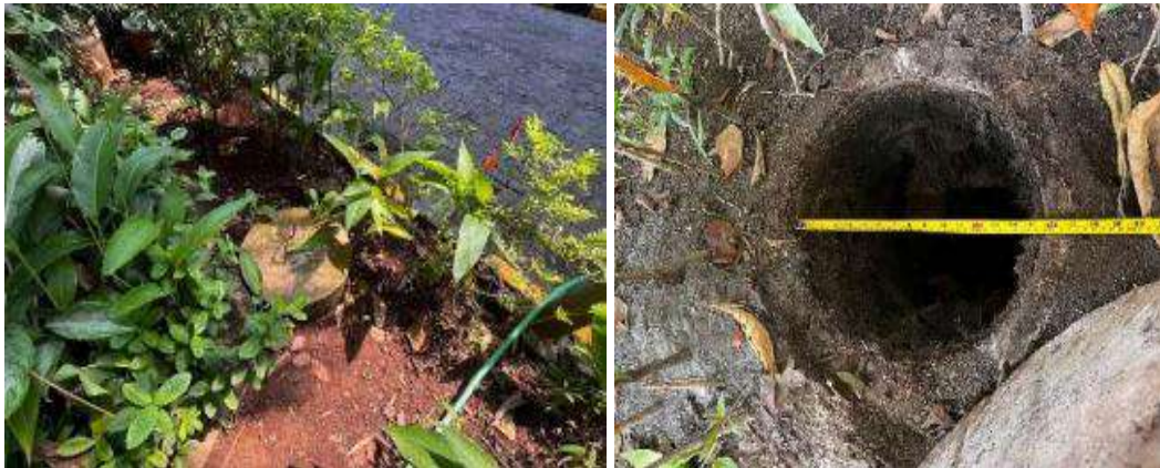
Preparation of Infiltration Wells
