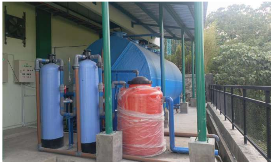
Bio Filter Reservoir on the Floor
