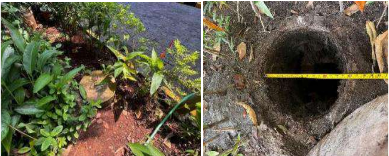
Preparation of Infiltration Wells
