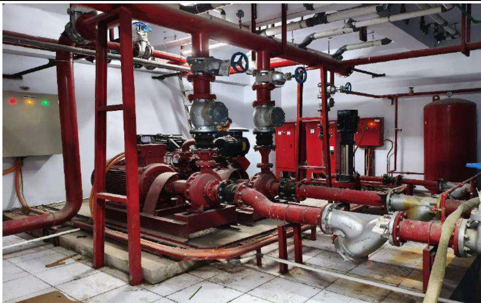
Hydrant Pump and Springler System
