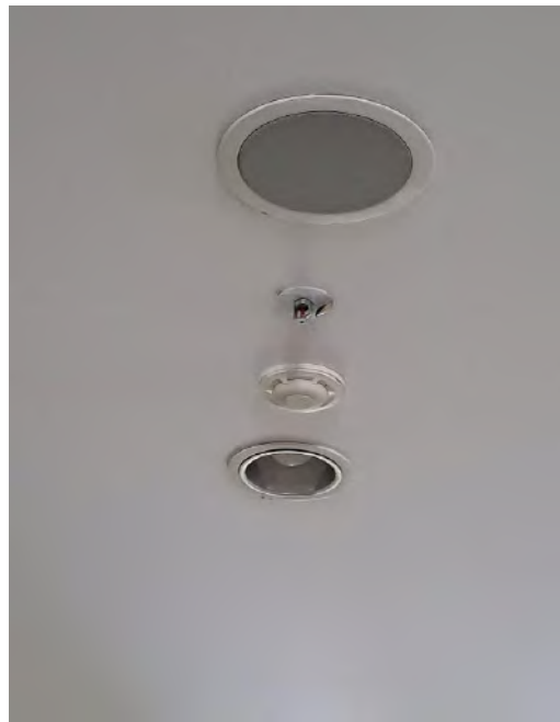
Smoke Detector, Springler and Speaker Paging
